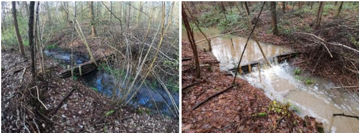
Figure 1 The same leaky woody dam during normal (left) and high (right) flow conditions.
